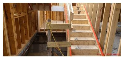
The front stair case framing is complete from basement to fifth floor we are working on the rear stair case now
