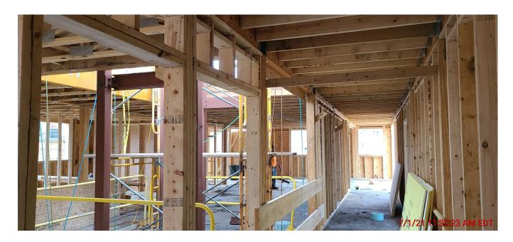
4th floor structural framing is complete. The steel in the picture are the supports for the elevator track system
