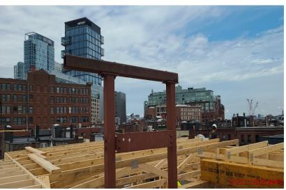
We are ½ way through roof framing the steel you see is for the elevator penthouse and hoisting beam that will be installed in the next few weeks
